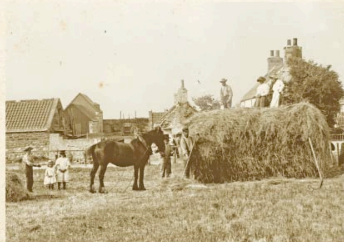
Dairy Farm, Cullen Street
