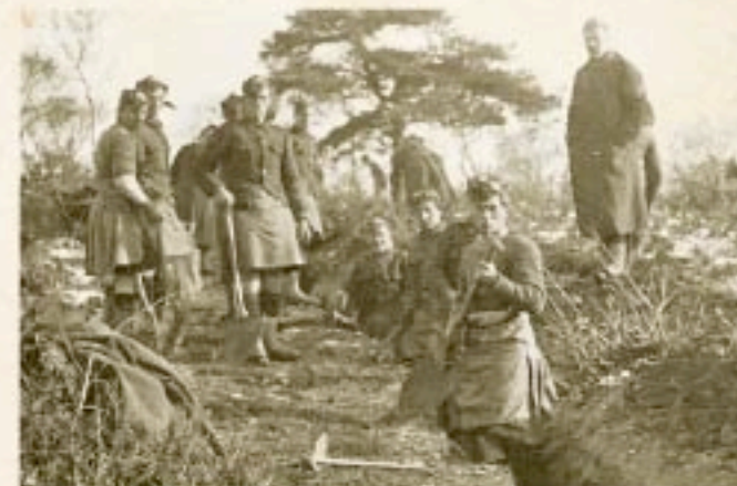
6th Gordon Highlanders digging trenches in France
